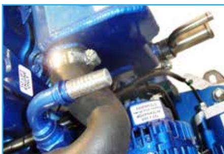
Hot water connections
