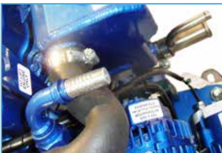
Hot water connections
